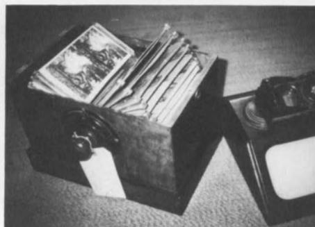
*Cadwell Viewer with top removed. Note views loaded facing both directions in holders. Collection of North Reading, MA Library.*
