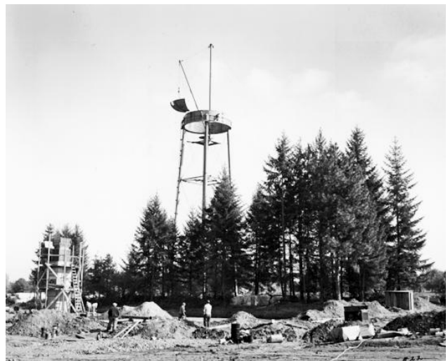
Above: Progress at Progress...the water tower goes up in early stage of construction.
